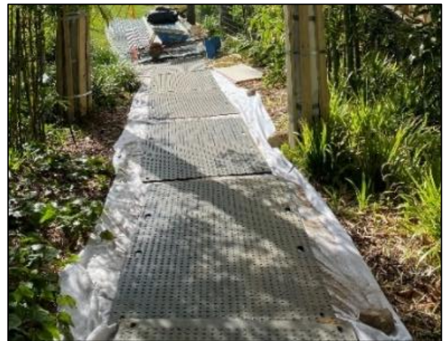
Figure 7: Spreader plates
