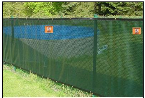
Figure 5: Supplementary fencing against existing fences.
